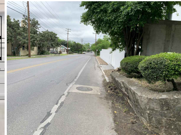
D STA. 4+70 M.H. C1 (#11622) (D.S. VIEW)
