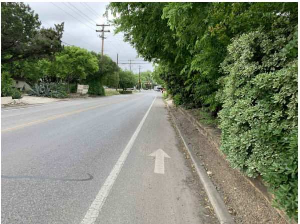
B STA. 2+00± POINT REPAIR AREA (D.S. VIEW)
