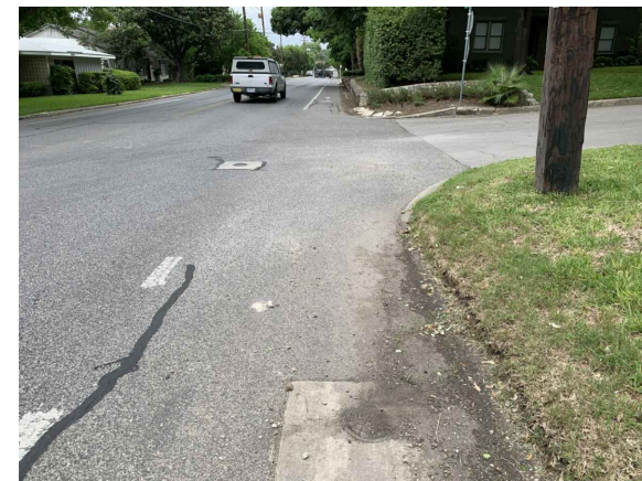
F STA. 6+70 WTR. VALVE (D.S. VIEW)
